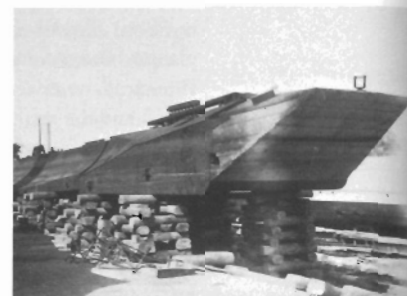
The pontoon for transporting U-boat parts along the Elbe and Danube en route to the Black Sea.
