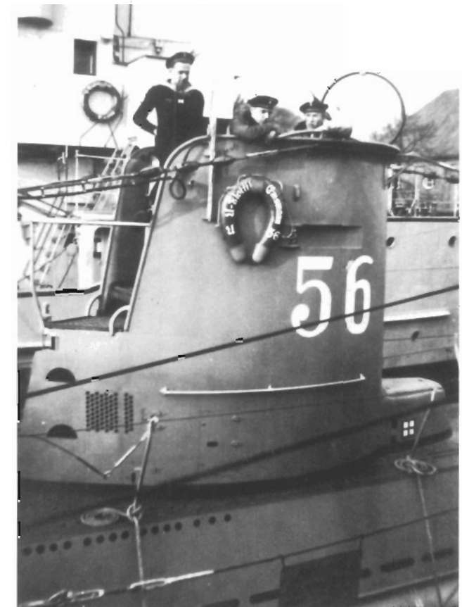
The typical early conning tower with sleek straight lines. This may have looked good, but the design was not terribly practical when it came to battering against heavy seas. The circular aerial of the radio direction finder can be seen by the elbow of the man on the right, and the white painted square with a cross (on the bulge by the base of the conning tower housing the magnetic compass) was an indicator to help potential rescuers in case of a diving accident. There were usually two of these. The square with the cross indicated an inlet for an emergency air supply for blowing the tanks without help from the crew. The other, a circle with a cross, marked an inlet for blowing fresh air into the interior. In addition to these two, it is possible to find some covers marked with an inverted 'T' indicating the fuel and oil inlets.
