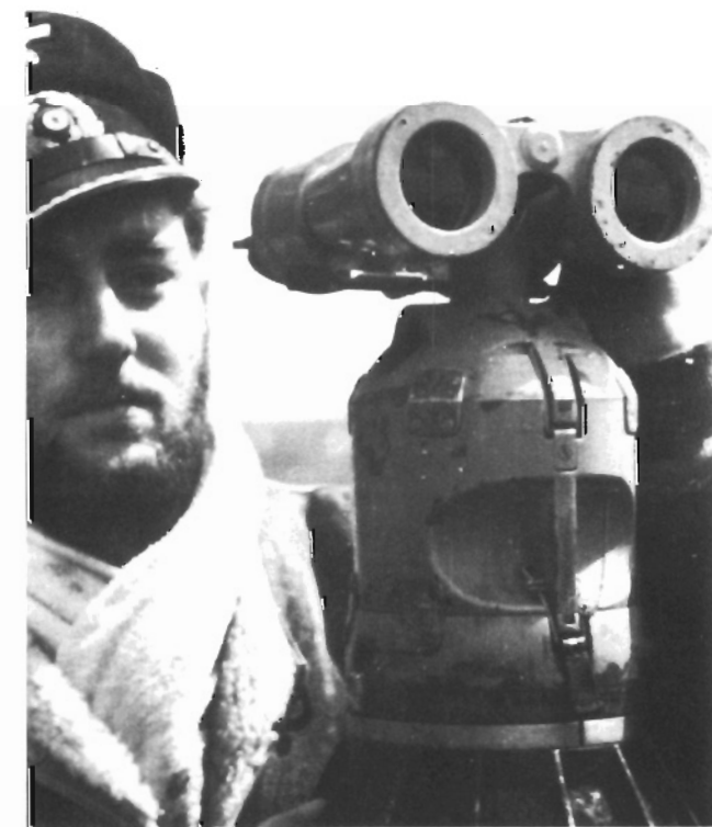
The UZO (U-Bootzieloptik), or U-boat Target Binocular, clipped in position on top of the torpedo aimer. Early in the Second World War, it was necessary to aim the entire boat at the target, but angle deflectors were soon fitted to make this difficult job much easier. During surface attacks, the commanders would stand back to keep an overall eye on the proceedings and tell the First Watch Officer which targets to aim at. The suggestion made by some historians that the commander was below in the central control room working a torpedo calculator is not true. Incidentally, there was no grid inside these special, water-resistant binoculars nor even an indication to mark the centre. Looking through them one saw the same plain circular view as one would get through normal glasses.
