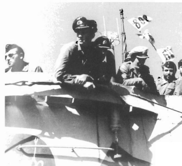
U593 under Kptlt Gerd Kelbling (wearing the white hat). To the left of the partly extended attack periscope is the newer dipole aerial for the Metox radar detector, which did not have to be dismantled every time the boat dived. This particular model was fitted quickly as a stop-gap measure. Later these devices were positioned so that they could be retracted into the conning tower wall.
