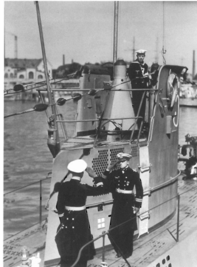
U51, an early Type VII B from Germaniawerft, showing the Wintergarten before the navy got around to supplying U-boats with proper anti-aircraft guns. At this time, in 1938, it was thought aircraft would not present a great threat, since submarines would dive before they came too close. This photograph was taken in the naval harbour at Kiel-Wik. The slightly blurred building in the background was still there at the beginning of the twenty-first century, although it looks as though the tall chimney may have been rebuilt after the war.
