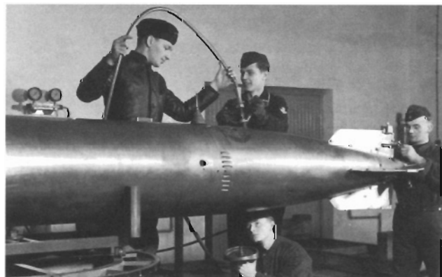
The tail end of a G7e torpedo. This had an advantage over the G7a in that it did not leave a noticeable trail of bubbles, but constant maintenance was necessary to keep the batteries charged to capacity. This photo was taken during a training session on land.
