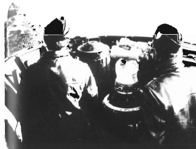
The UZO (U-Bootzieloptik), or U-boat Target Binocular, clipped in position on top of the torpedo aimer. Early in the Second World War, it was necessary to aim the entire boat at the target, but angle deflectors were soon fitted to make this difficult job much easier. During surface attacks, the commanders would stand back to keep an overall eye on the proceedings and tell the First Watch Officer which targets to aim at. The suggestion made by some historians that the commander was below in the central control room working a torpedo calculator is not true. Incidentally, there was no grid inside these special, water-resistant binoculars nor even an indication to mark the centre. Looking through them one saw the same plain circular view as one would get through normal glasses.
